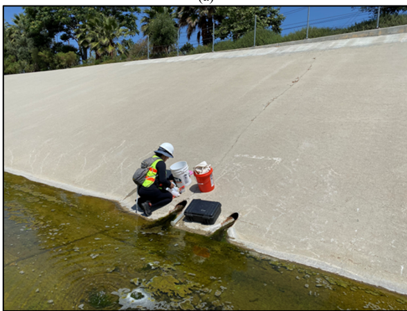
Fig. 19. Groundwater-surface water interactions in the Los Angeles River: (a) Cross section of the Los Angeles River shows channel flow direction and groundwater seepage locations along the concrete lining within a shallow aquifer; (b) groundwater seepage along the concrete lining located in the Upper Los Angeles River.
