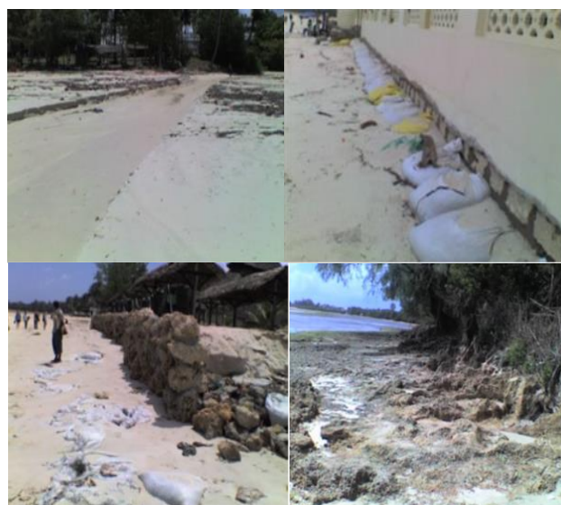
Fig. 3. Some of photos showing erosion activities at Bamburi beach.
