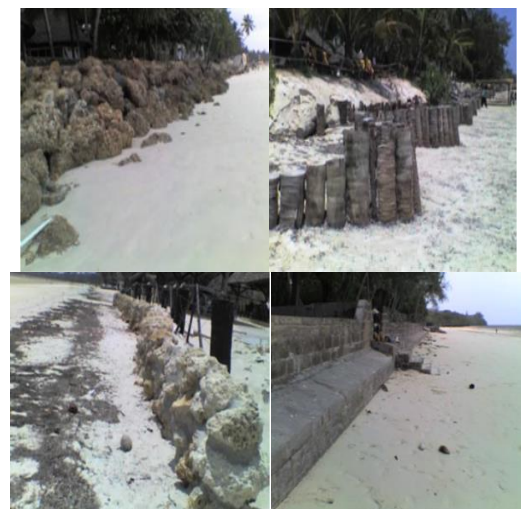
Fig. 1. Some photos showing shoreline protection measures at Bamburi beach.
