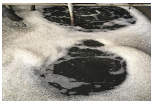
Fig. 5. AERATE stage with incomplete detergent destruction in DESTRUCTION stage.
