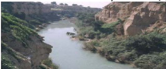
Fig.2 Stone and rocky walls of the Gar-Gar
