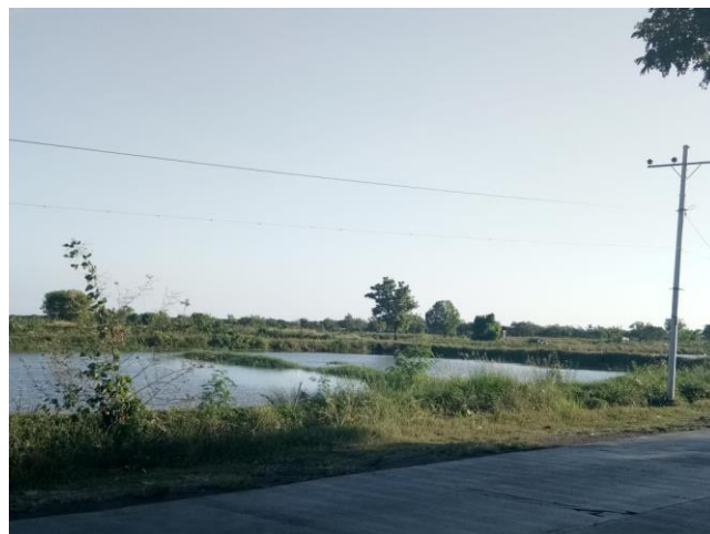
Fig. 8. Salt-pond alongside to Biringkassi power plant.
