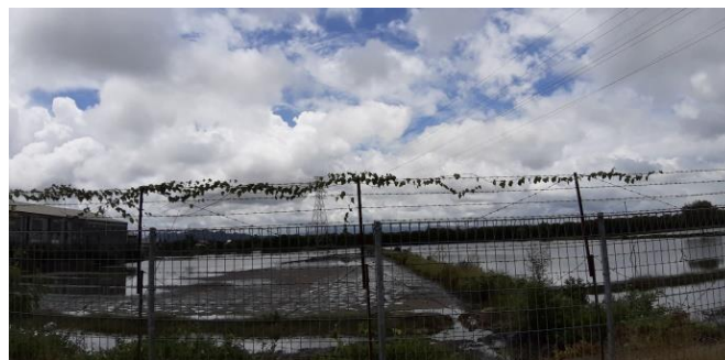
Fig. 7. Salt-pond by the side of Biringkassi power plant.
