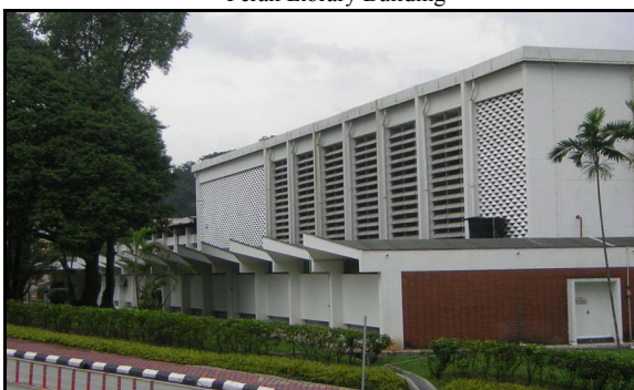
Pic 2: Hung Louvers a Shading Tool at the West Side of UM Main Library Building
