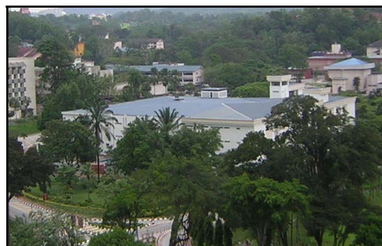
Pic 4: Landscape at the entire view of UM Main Library Building.
