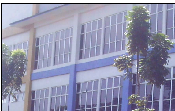
Pic 1: There is no Shading Tool at the Window of UiTM Perak Library Building
