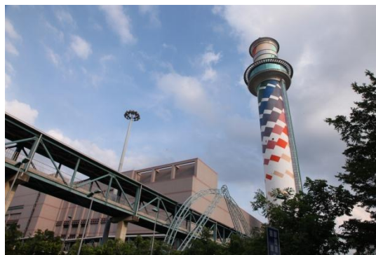
Beitou Refuse Incineration Plant
